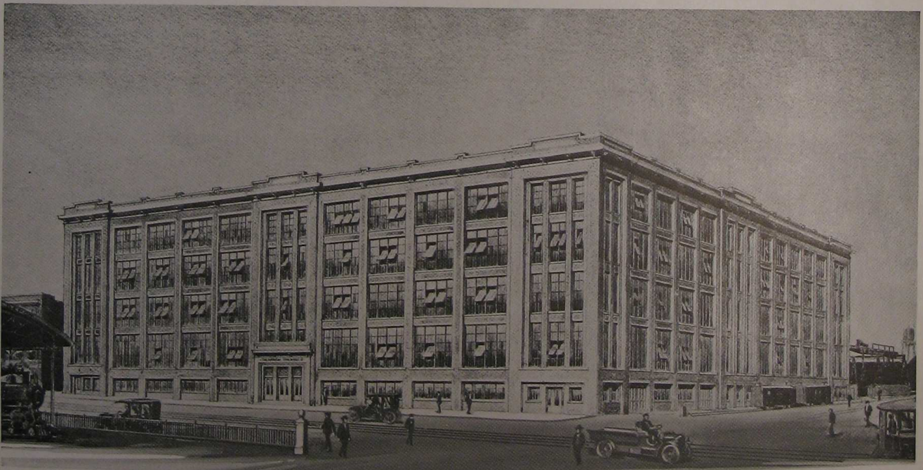
FIVE STORY BUILDING, RE-INFORCED CONCRETE CONSTRUCTION, ABSOLUTELY FIRE-PROOF — PROVIDES IDEAL WORKING SURROUNDING — 245,000 SQUARE FEET OF FLOOR SPACE.
