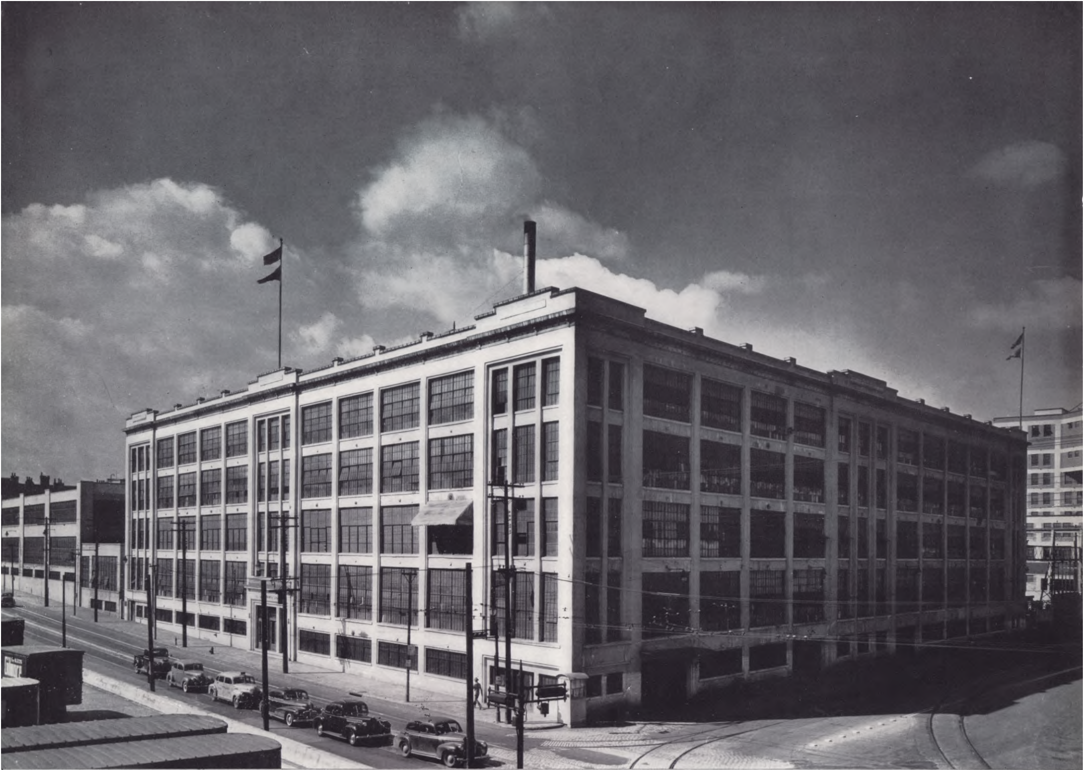
Plant of The American Tool Works Co., Cincinnati, Ohio. Floor Space, 365,500 square feet. Number of employees at capacity, 1600
